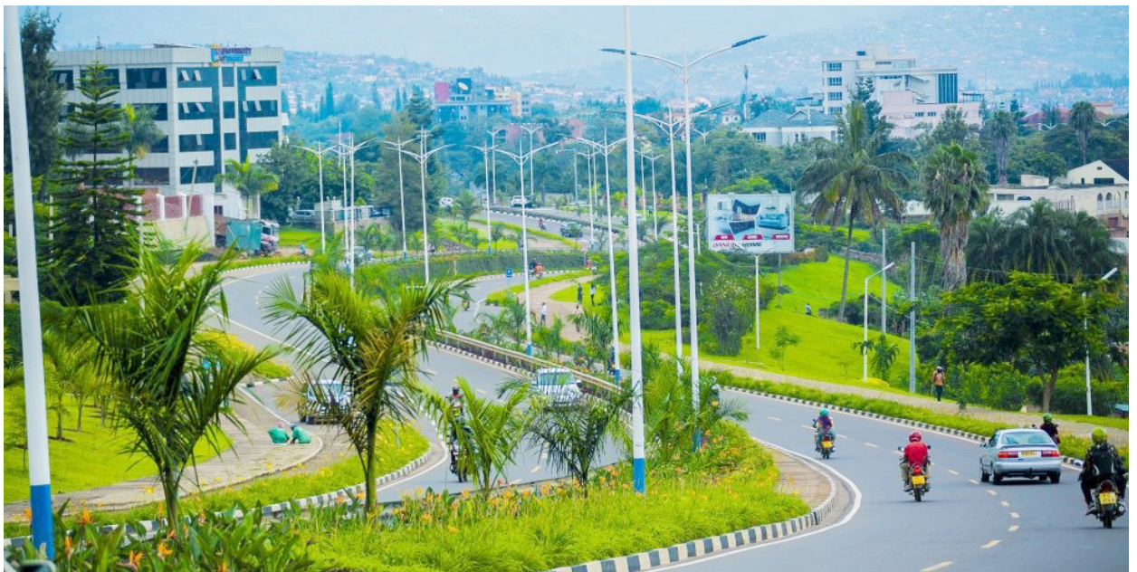
One of the many roads built by China Road & Bridge Corporation Limited. Photo: (Courtesy)
