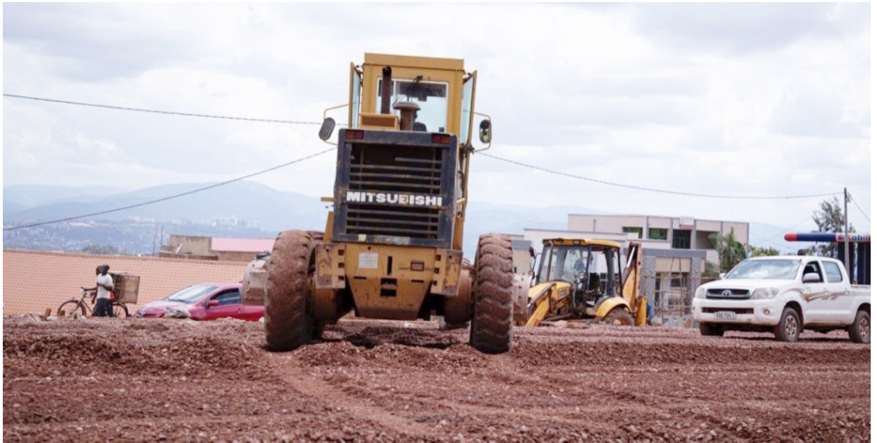
CRBC road construction works at Kicukiro-Kigali. Photo: Africa China Review
