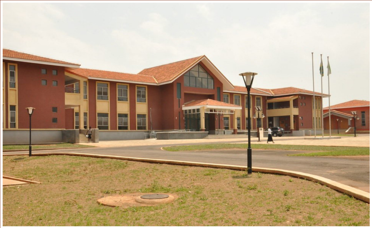
IPRC Musanze campus after renovation
